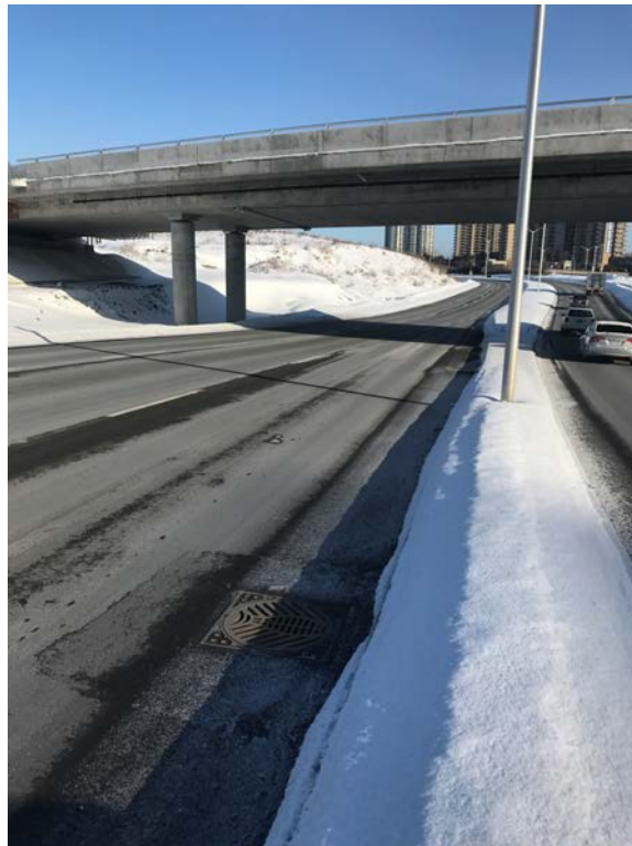
Old pavement markings grinded out along southbound Riverside Drive from south of Frobisher to south tie-in
