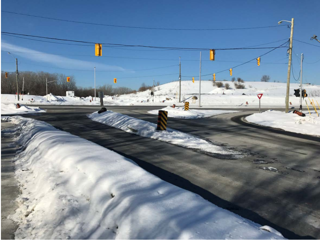
Hazard marking signage installed at Hincks and Riverside intersection
