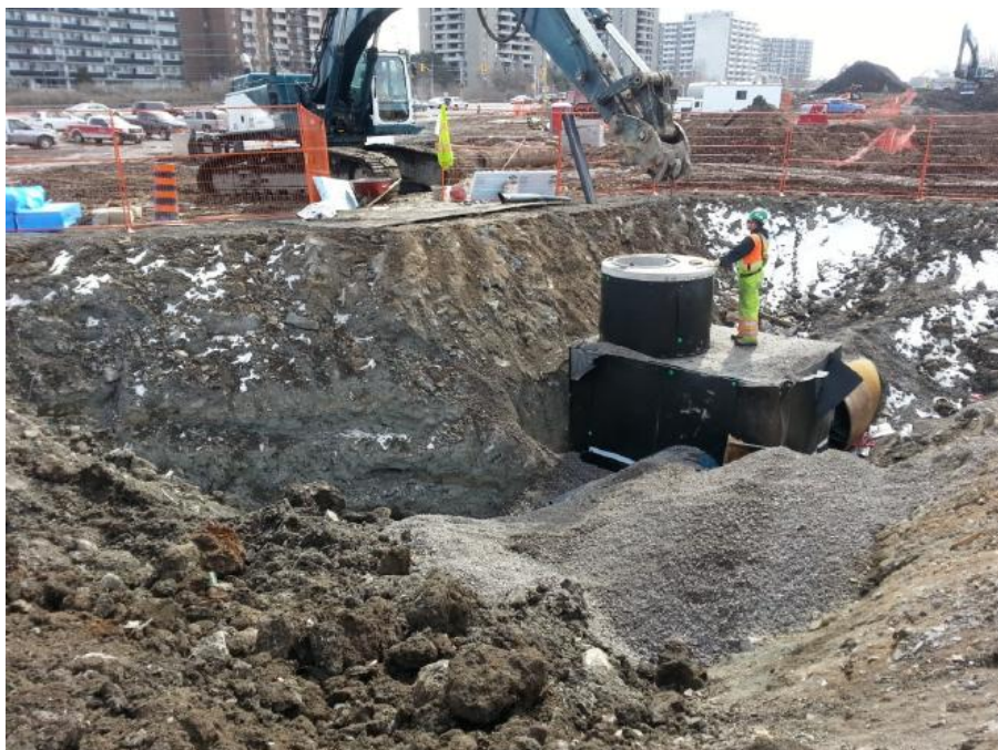
914mm diameter feedermain valve chamber
