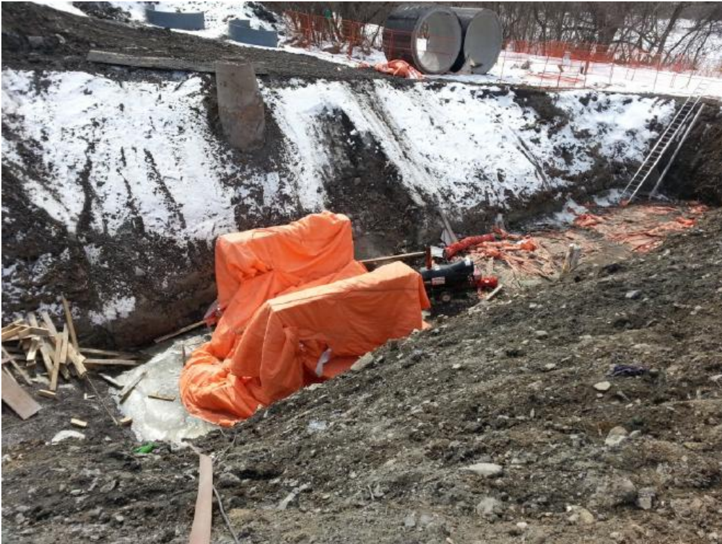
Storm Sewer installation including sanitary sewer crossing
