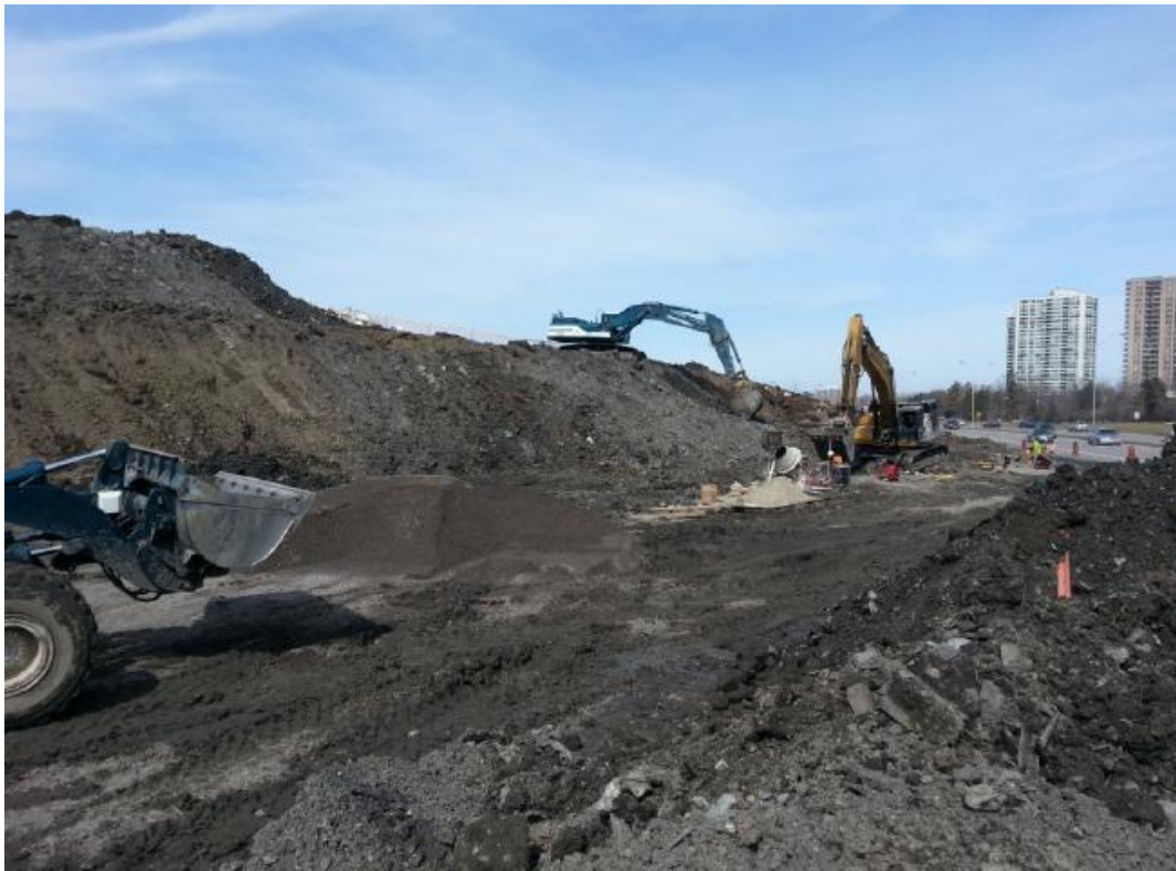
Excavation for realigned Riverside Drive
