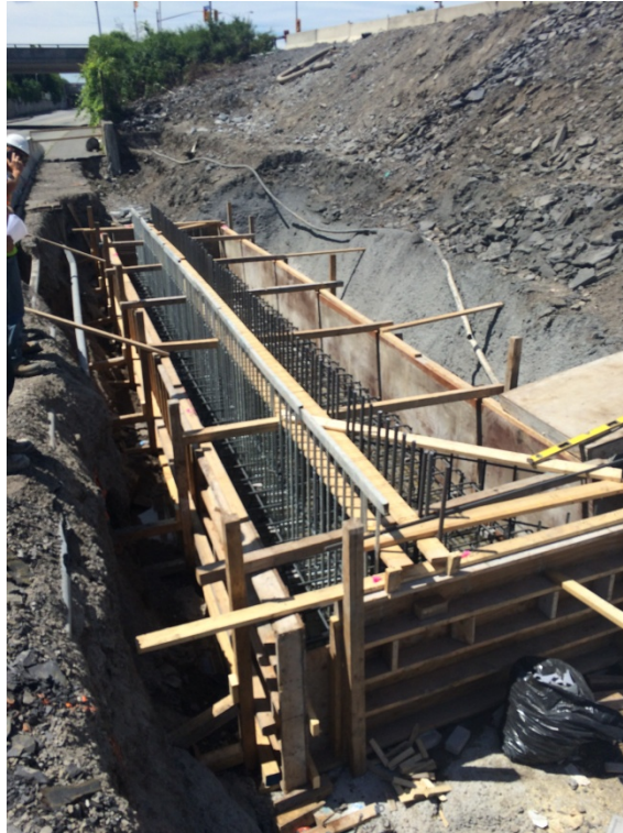
Rebar placed for Transitway structure west abutment footing.
