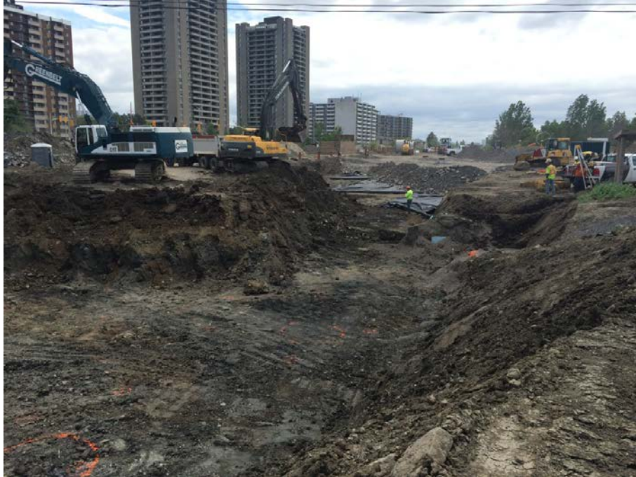
Excavation for realigned Riverside road.
