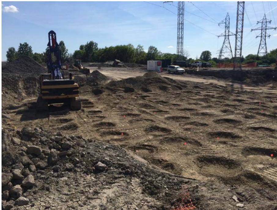
Rapid impact compaction for Riverside structure deck falsework.
