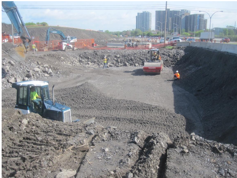
Engineered fill for Riverside Bridge East Abutment– May 26, 2015.
