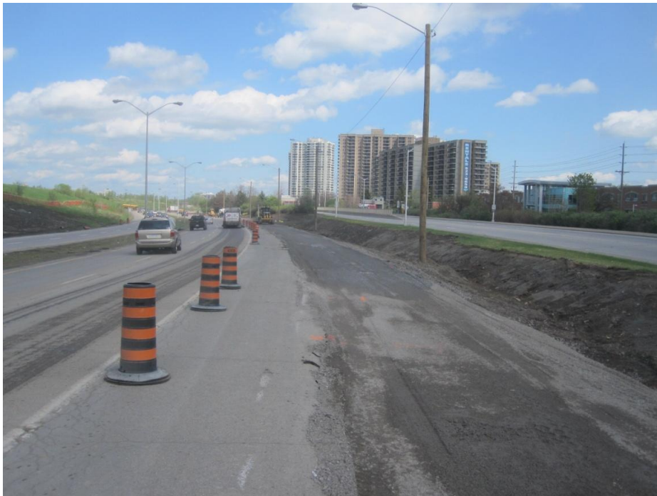
Grading of Riverside Drive Detour Widening – May 12, 2015.
