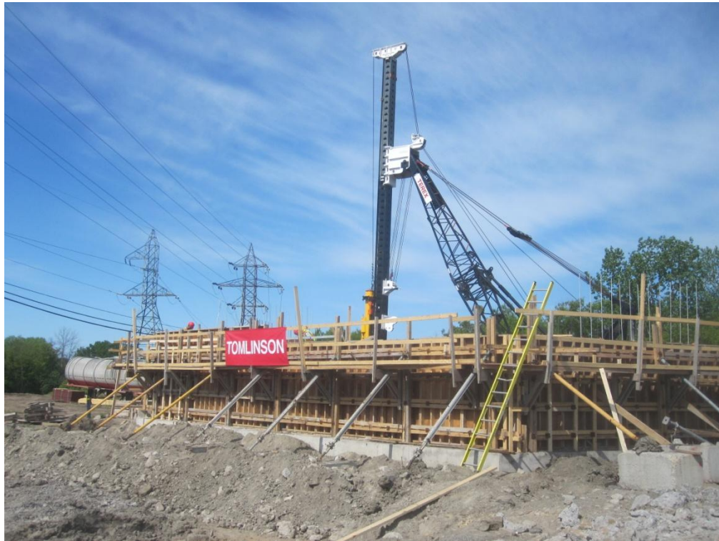
Riverside Drive Structure West Abutment Formwork – May 21, 2015
