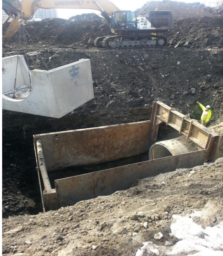
Large diameter Storm Sewer installation – April 8, 2015
