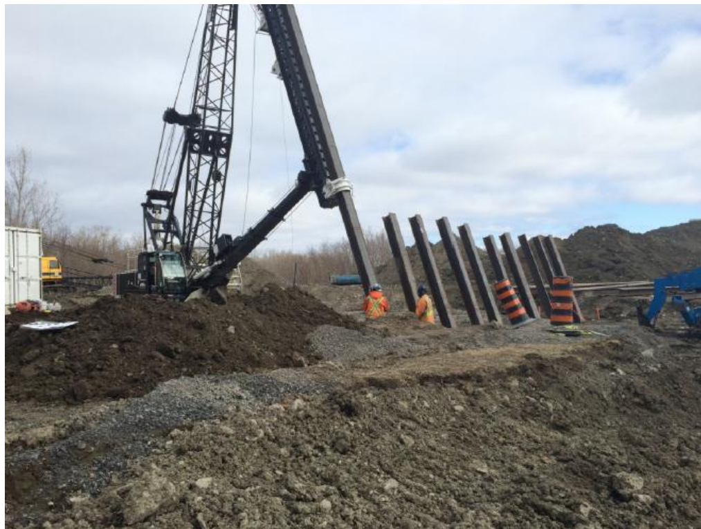
Piling for new Riverside Drive bridge foundations – April 25, 2015
