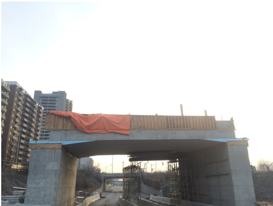
Construction of the Transitway structure bridge.
