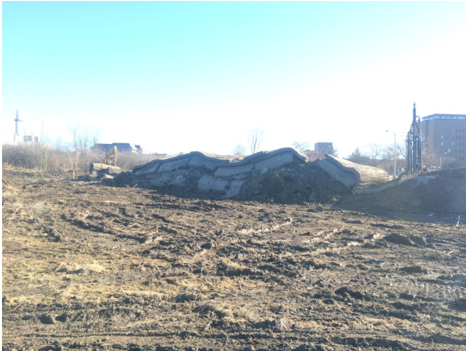
Controlled blasting of rock for storm sewer trenches.
