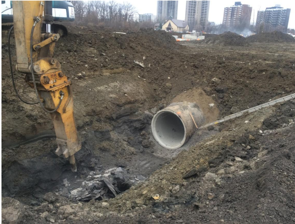
Installation of large diameter storm sewer to the east of Alta Vista Drive.
