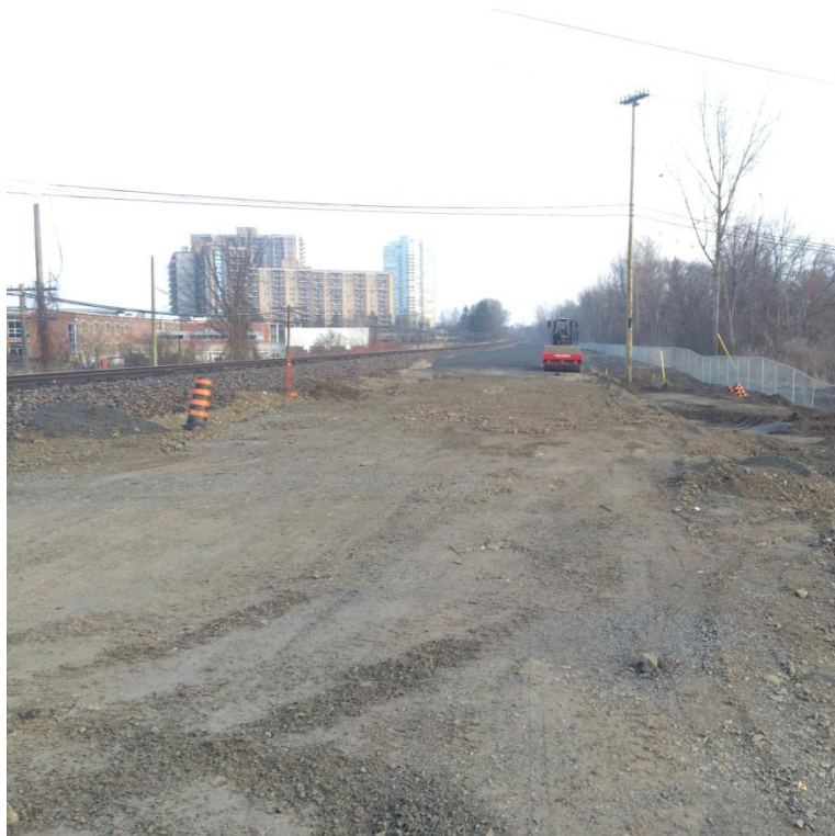
VIA rail temporary diversion embankment and backfilled post tensioned culvert.
