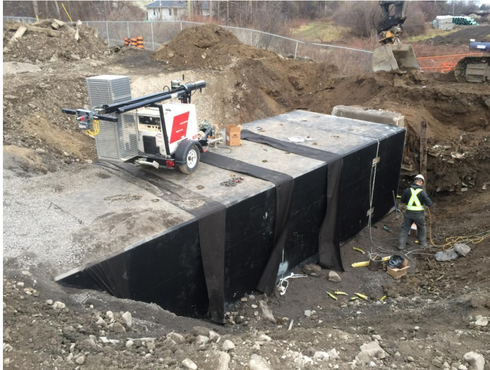
Installation of diversion portion of VIA rail post tensioned culvert.
