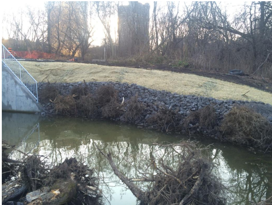
Moses Pepper Drain outlet showing embankment revetment.
