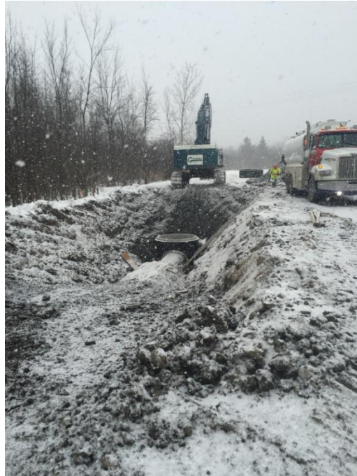
Installing storm sewer along the Hospital Link, east of Alta Vista.
