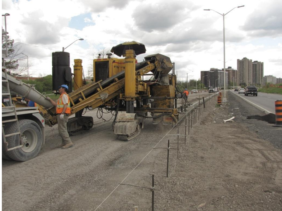
Placing curb along northbound Riverside.
