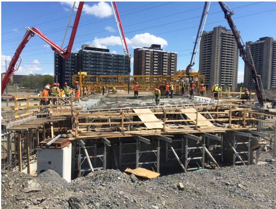
Pouring Riverside structure deck.
