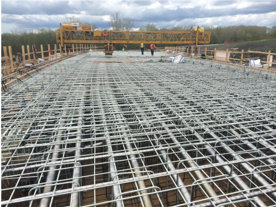
Rebar and post tensioning for the Riverside structure deck.
