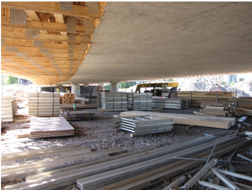
Removing formwork and falsework from Riverside structure deck.
