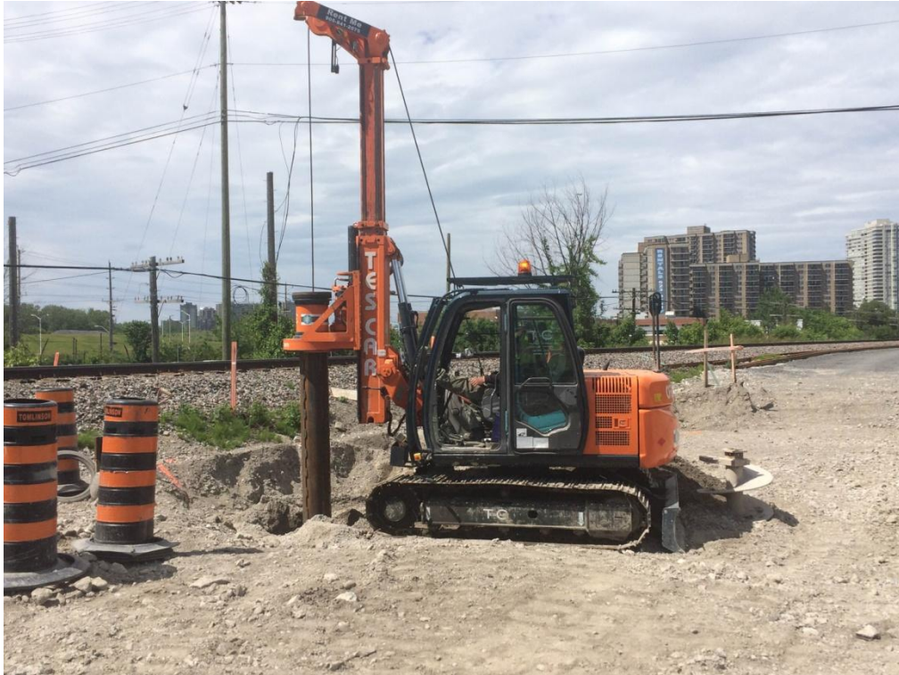
Drilling for VIA shoring wall.
