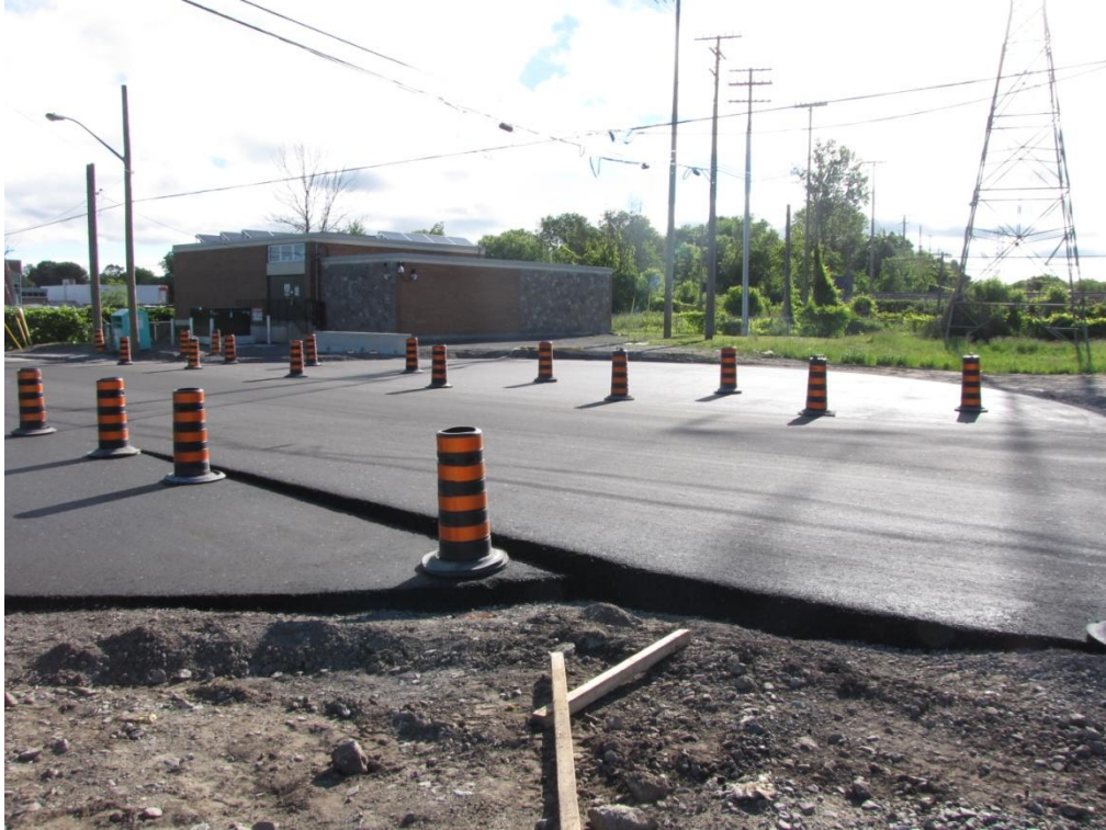
North cul-de-sac on Old Riverside paved, with temporary ramp for Old Riverside while it is still open.
