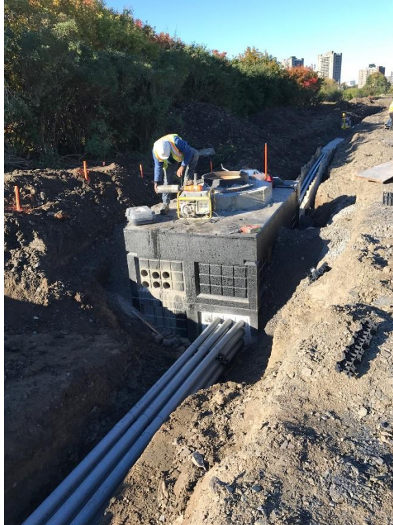
Installation of new Hydro Ottawa duct bank structure along the Hospital Link.
