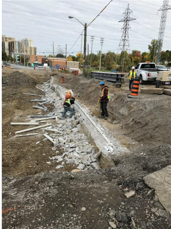
Removing an existing duct bank structure along Old Riverside.
