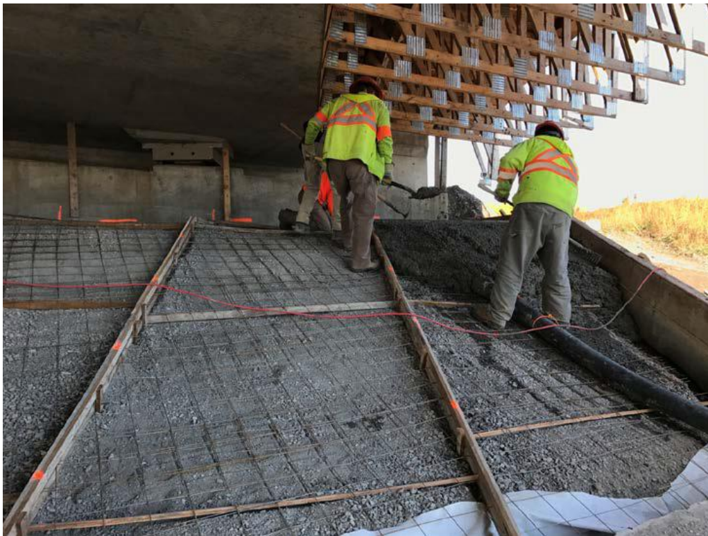
Pouring concrete for Riverside structure slope paving.
