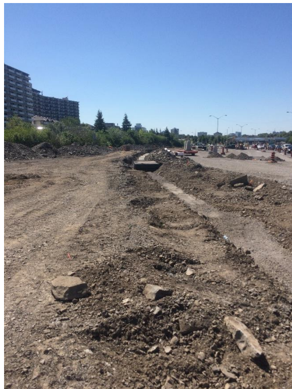
New Hydro duct and maintenance hole installed along the east side of realigned Riverside Drive.
