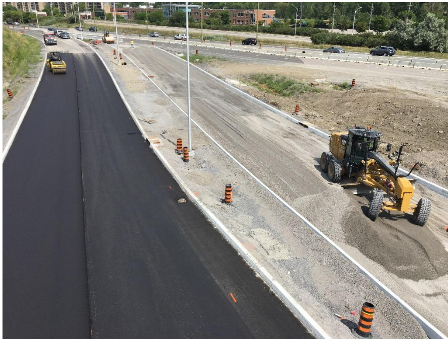
Paving and grading of realigned Riverside Drive, north of the Riverside structure.
