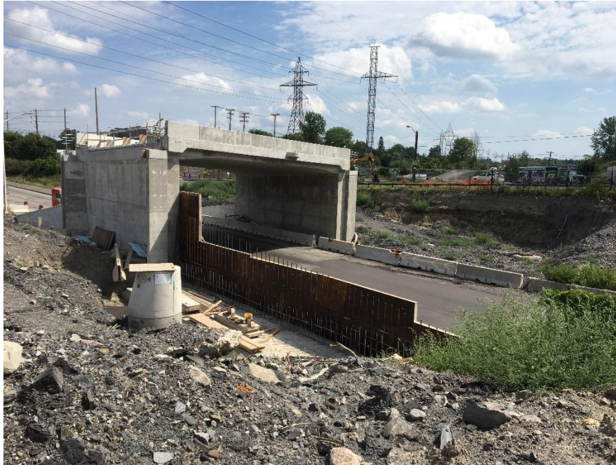
Construction of the southwest Transitway retaining wall.
