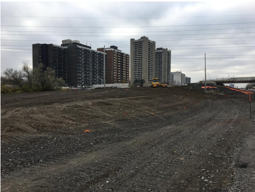
Grading and shaping berm along east side of Realigned Riverside Drive (shown north of Riverside Structure)
