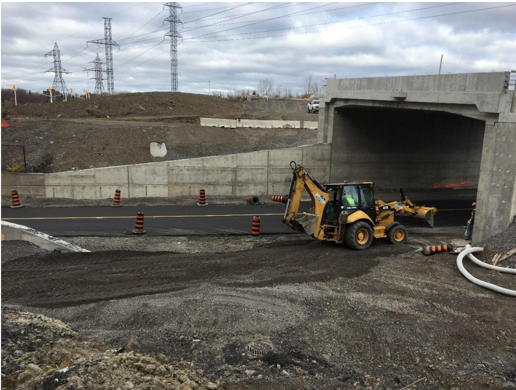
Grading of Granular 'B' along east side of Transitway
