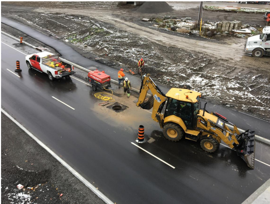
Adjusting manholes in the northbound lane of Realigned Riverside Drive.
