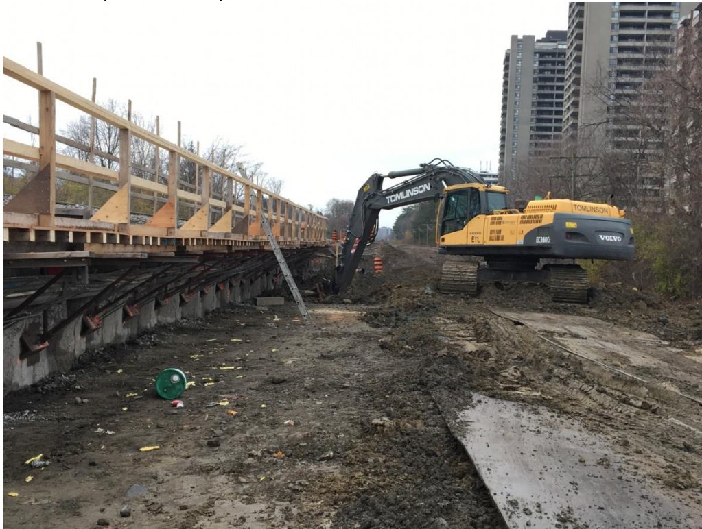
Excavating for second row of tie-backs against shoring wall in VIA corridor
