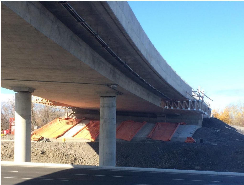
Concrete placed in slope paving at Riverside Structure (west shown)
