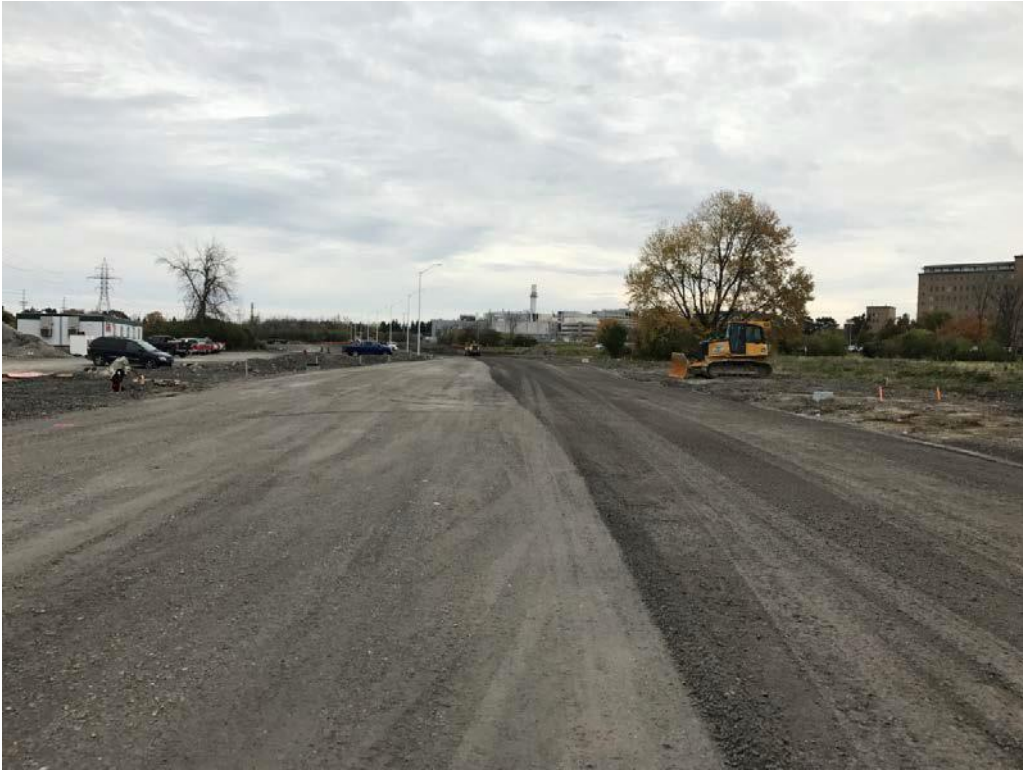
Fine grading and compaction of Granular material for Link Road east of Alta Vista
