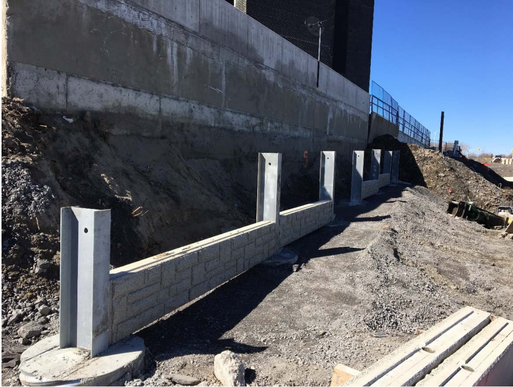
Construction of the narrow Footprint Durisol Wall.
