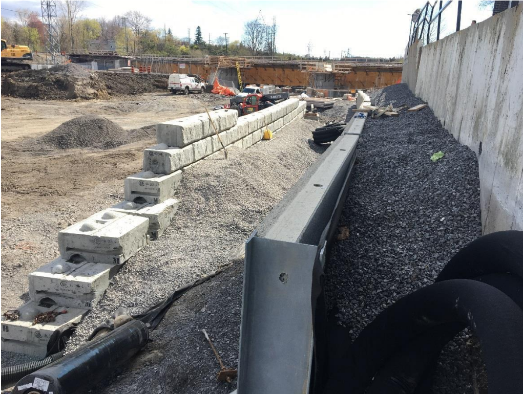
Stone blocks and granular material placed along future Hospital Link roadway west of VIA corridor.
