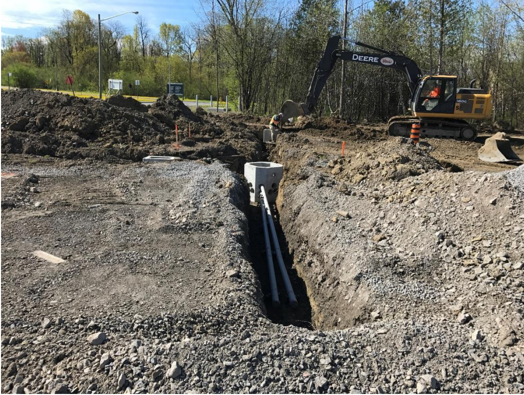
Installing traffic and streetlighting plant west of Alta Vista for future Hospital Link intersection.
