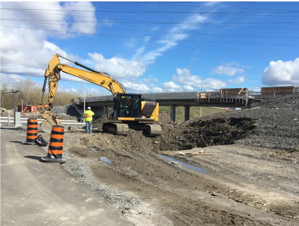
Excavation to repair existing watermain on Frobisher and Riverside Intersection.
