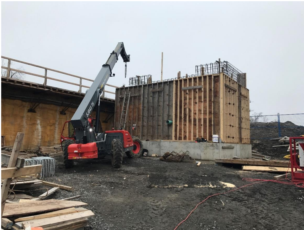
Forming and bracing south abutment and wingwalls.
