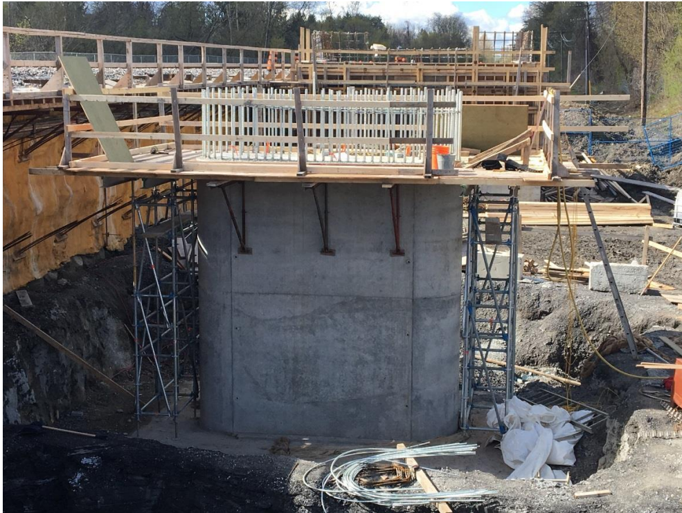
Construction of south pier and pier cap at VIA structure.
