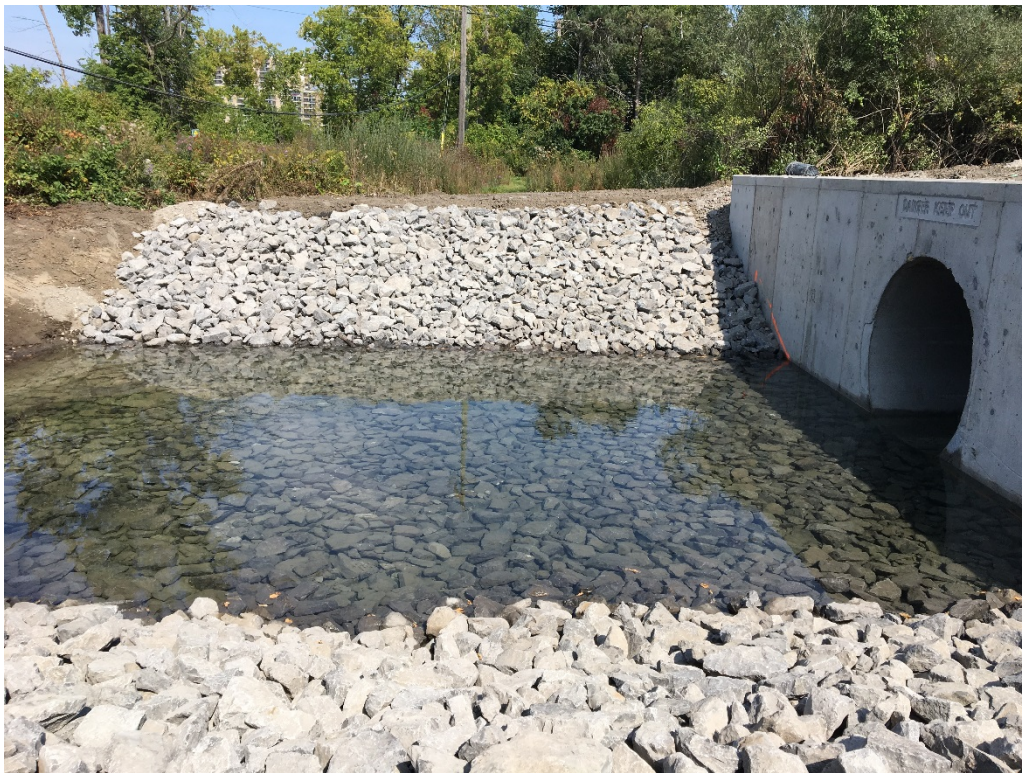
Construction of Hospital Link outlet with concrete headwall and riprap protection
