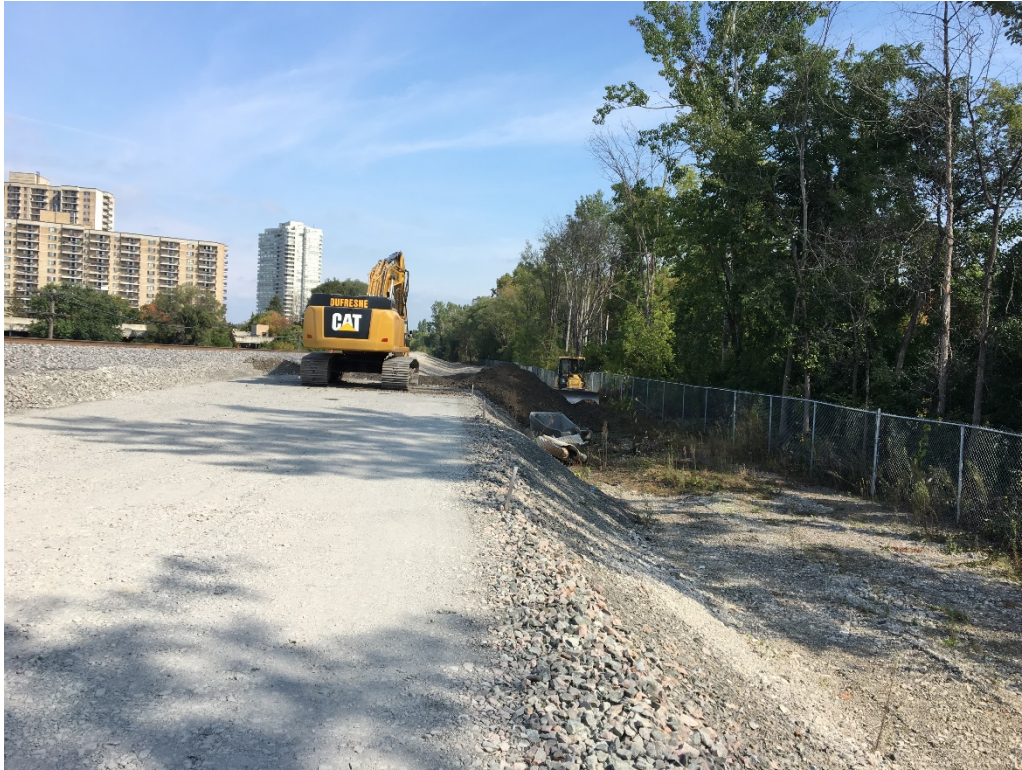
Removal of diversion track sub-ballast
