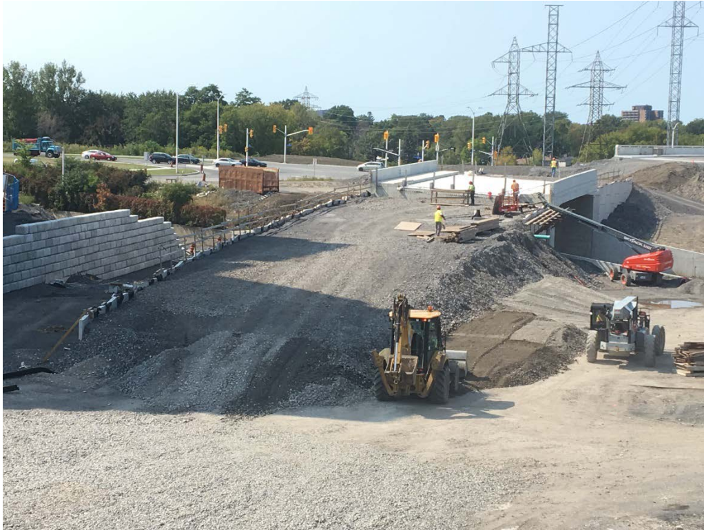
Retaining walls and grading on east side of Transitway structure
