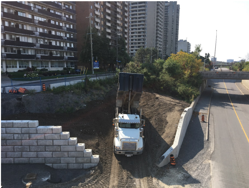
Grading for the south cul-de-sac on Old Riverside Drive
