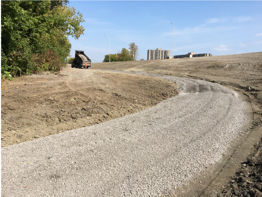
Grading of MUP west of Riverside Structure toward Rideau River pathway
