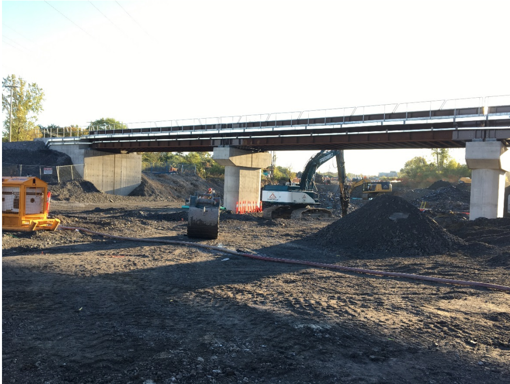
Construction of the Hospital Ring Road under the VIA structure
