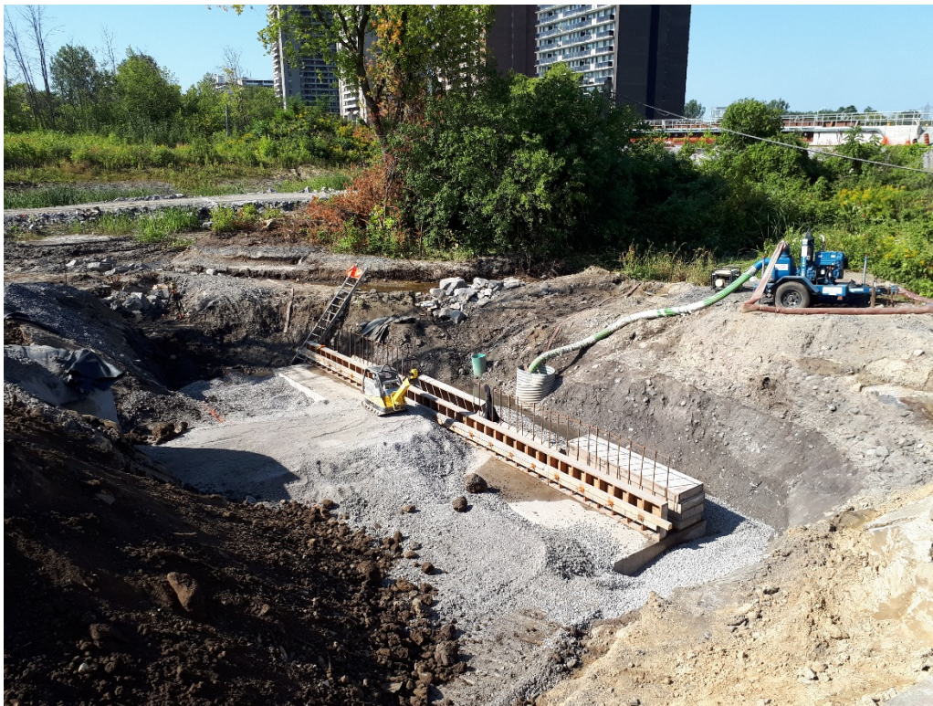
Construction of Hospital Link outlet headwall
